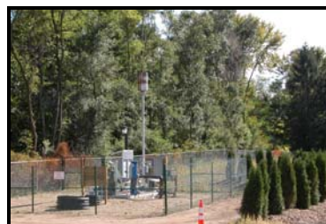
Design/Build and Installation of LFG Flares w/ PLC and Telemetry Uplink Systems
